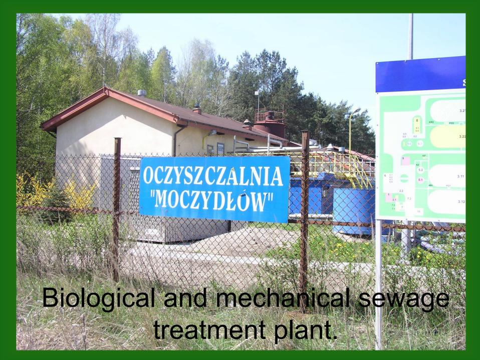
In our Moczydłowie we have a biological and mechanical sevage treatment plant. The sevage is first purifiet mechanically and then biologically treatet. The sediment and sludge left over after the sludge process of the biological purification (biofiltration) is recycled as manure for the surrounding land area. There are no chemicals used in this treatment plant. The water is sent to back to the homes in our area.
